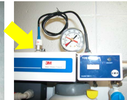
Adjust blending via needle valve
