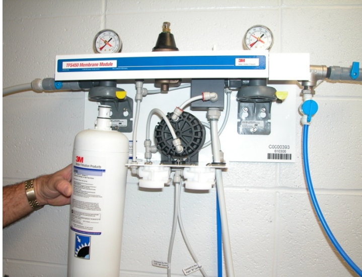
Pre-Filter installation
