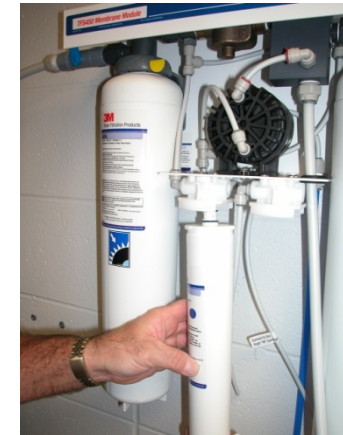
Install RO ctg
