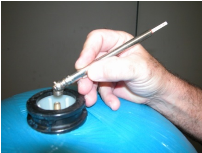
Adjust tank air
