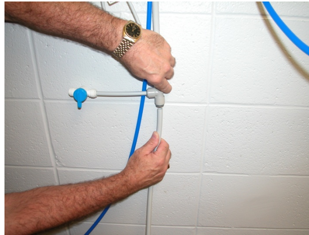
Install tank line sample valve
