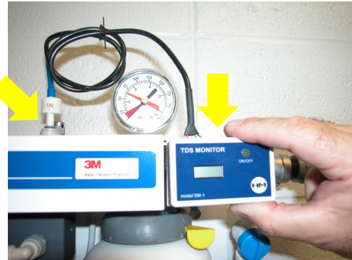
Mount TDS Monitor and Insert TDS probe
