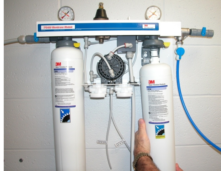
Post-Filter installation
