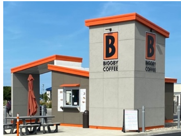
Figure 2: EnduraWal Dryvit) Exterior
